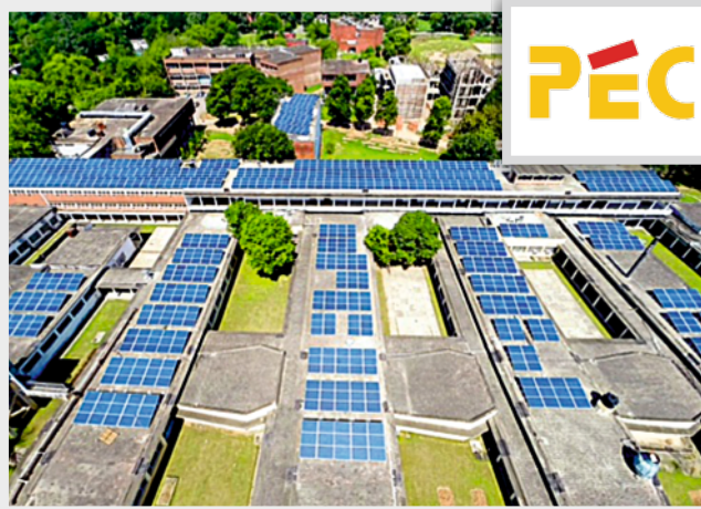
1 MW Power India's Largest Grid Connected Rooftop Solar Plant on an Educational Institute - Punjab Engineering College, Chandigarh
